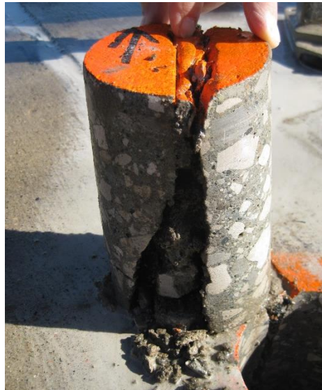
Figure 58. Core sample 4 from the distressed joint
