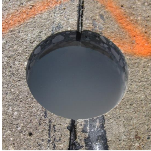
Figure 59. Field observation of impermeable subsurface below pavement (2 hours after test completed)
