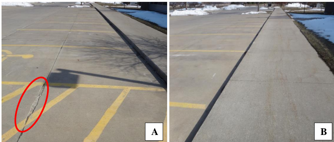
Figure 42. Field observation showing sidewalk performances better than parking lot (A: distressed parking lot, B: undamaged sidewalk)
