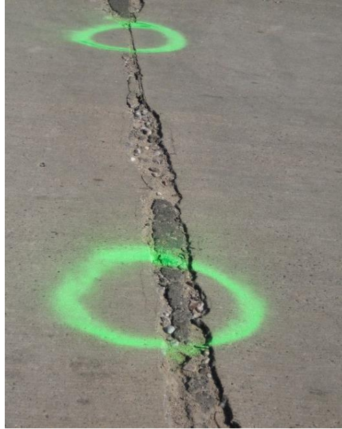
Figure 78. Grand Avenue in Eau Claire, Wisconsin
