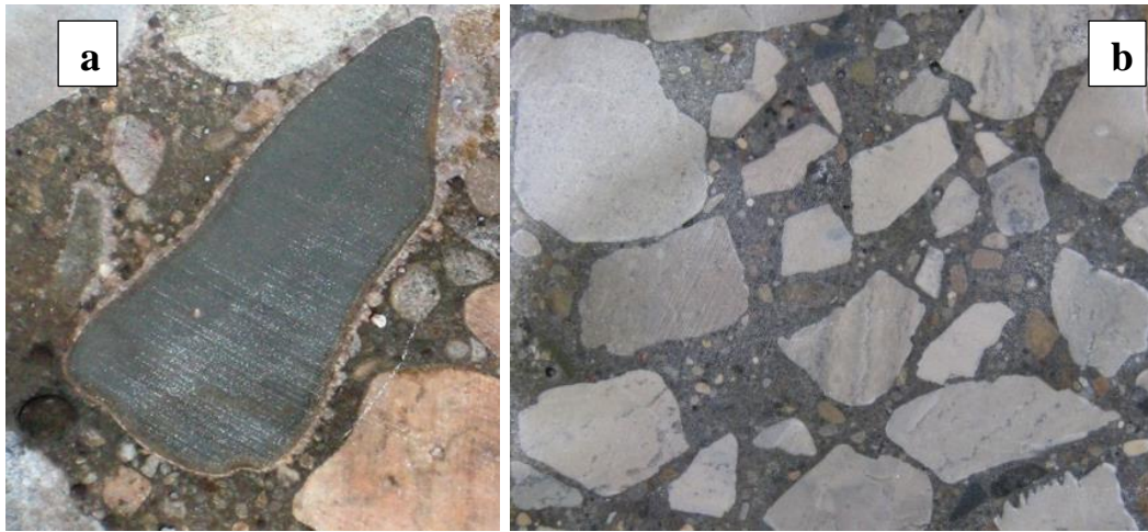
Figure 34. Silver nitrate sprayed samples for mapping chloride (a: concrete mixture using gravel; b: concrete mixture using limestone)
